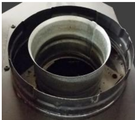
Vent Attachment Inspection – unbent and attached rings
