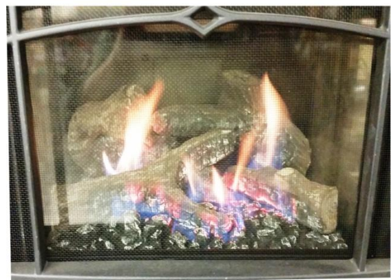
Figure 40 – Typical Burner Flame Appearance
