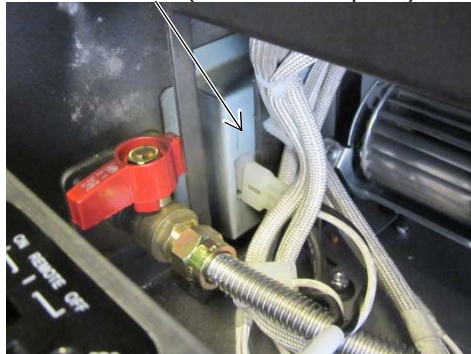
Junction Box (from inside fireplace)
